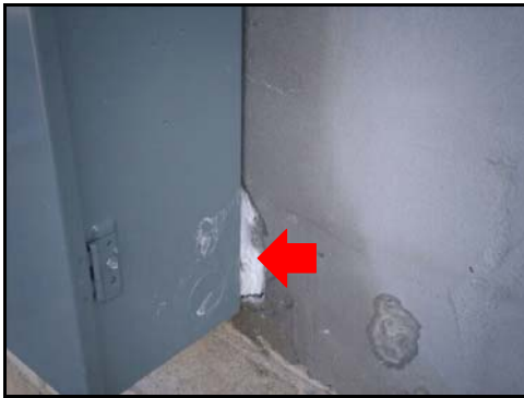
(7) Address gaps in block walls with mortar.
