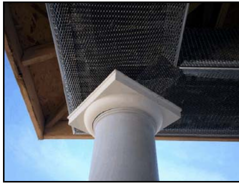
(3) Make sure column caps are square and centered at final install.
