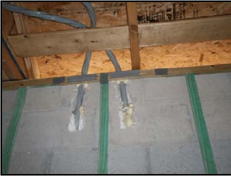
(11) Lintel block “chiseled” to accommodate the main electrical service cables.
