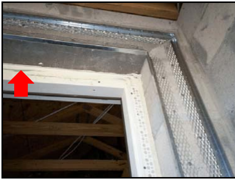
(2) After adjustments are made to the front door, reseal the jamb.
