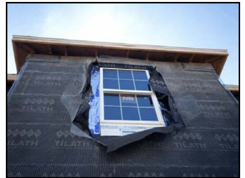
(10) Finish the stucco lath around the front 2 nd floor window.
