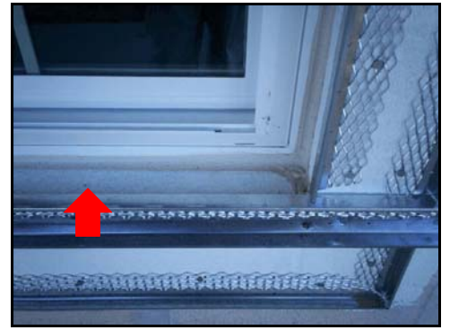
(4) Make sure finished window sills have slope.
