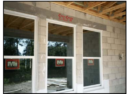
(6) Install stucco corner bead around rear windows.
