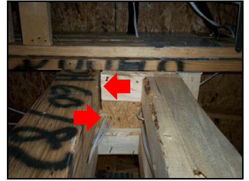
(13) Foam the voids in the wall cavities (draft stops throughout)
