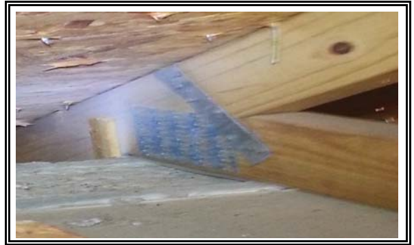
Roof to wall attachment -
