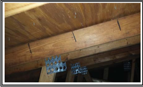
Roof deck attachment -
