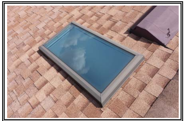
DOCUMENTATION PHOTO 2 SKYLIGHT
